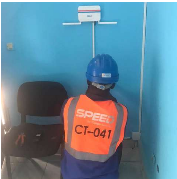
A technician from Congo Telecom doing the installation.
