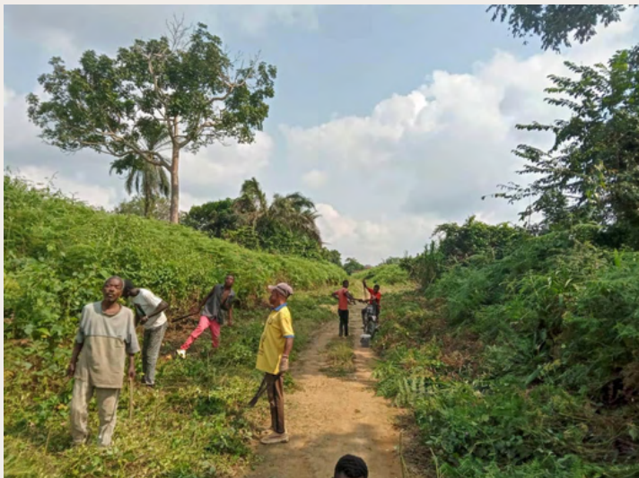
We cleared a secondary road that connects the two neighborhoods.
